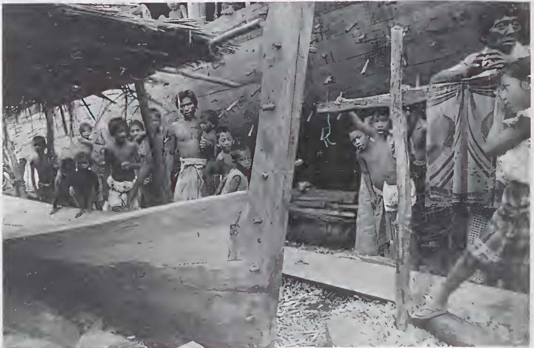
Fig. 19. Construction of a soppe at Mola (photo by Kurt Stenross).
